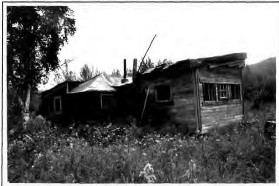
Figure 125. The Marcell/Dahl/Stevens/Friend/Olsen House, 1993. The view is looking northwest.
